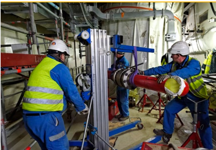
Mechanical installations on the Flamanville EPR site in 2014
