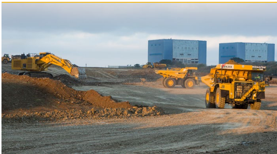
Preparatory works on the Hinkley Point C site in 2015
