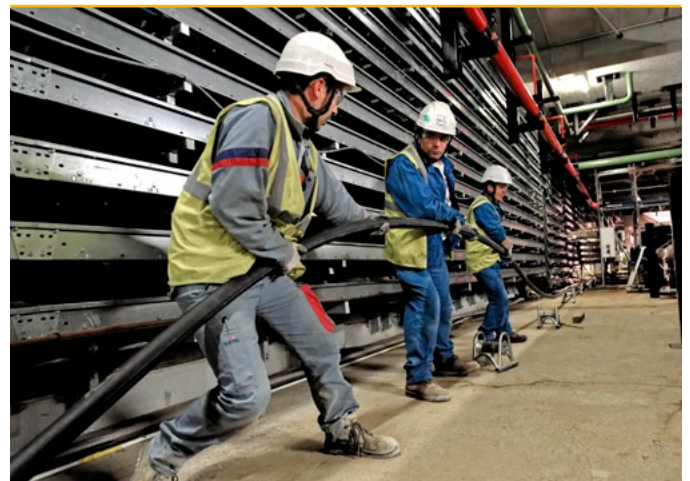
Electrical installations on the Flamanville EPR site in 2014
