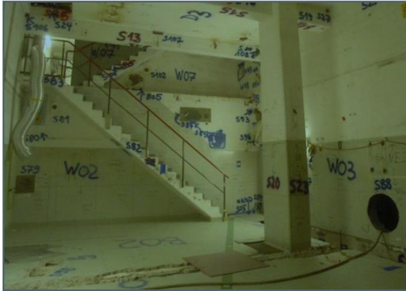
Figure 6: Room to be measured for clearance with sampling points (PreussenElektra GmbH, Würgassen nuclear power plant)
